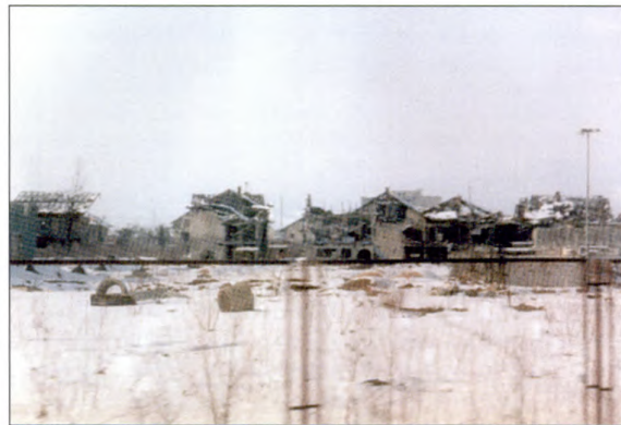
Damaged houses near Sarajevo Airport, as seen in 1996.
