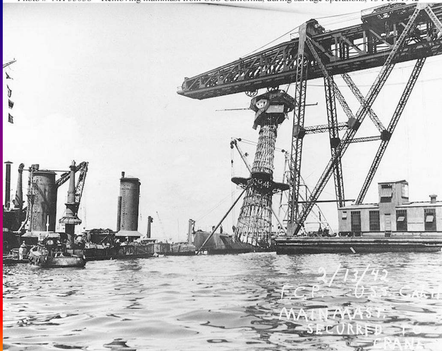
Photo # NH 55038 Removing mainmast from USS California, during salvage operations, 13 Feb. 1942
