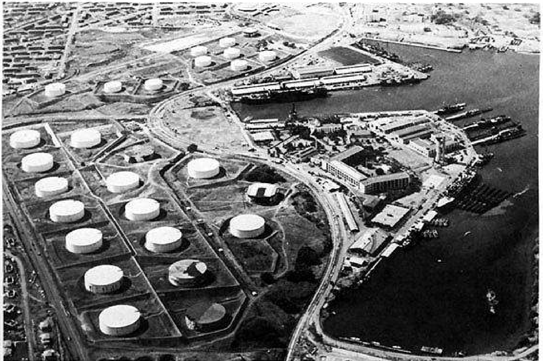
The submarine base and oil storage tanks on Oct. 13, 1941. None of these facilities were bombed, a fatal mistake for the Japanese.
