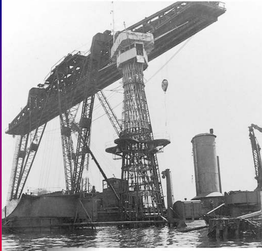
Photo # NH 55037 Removing USS California's mainmast, Feb. 1942
