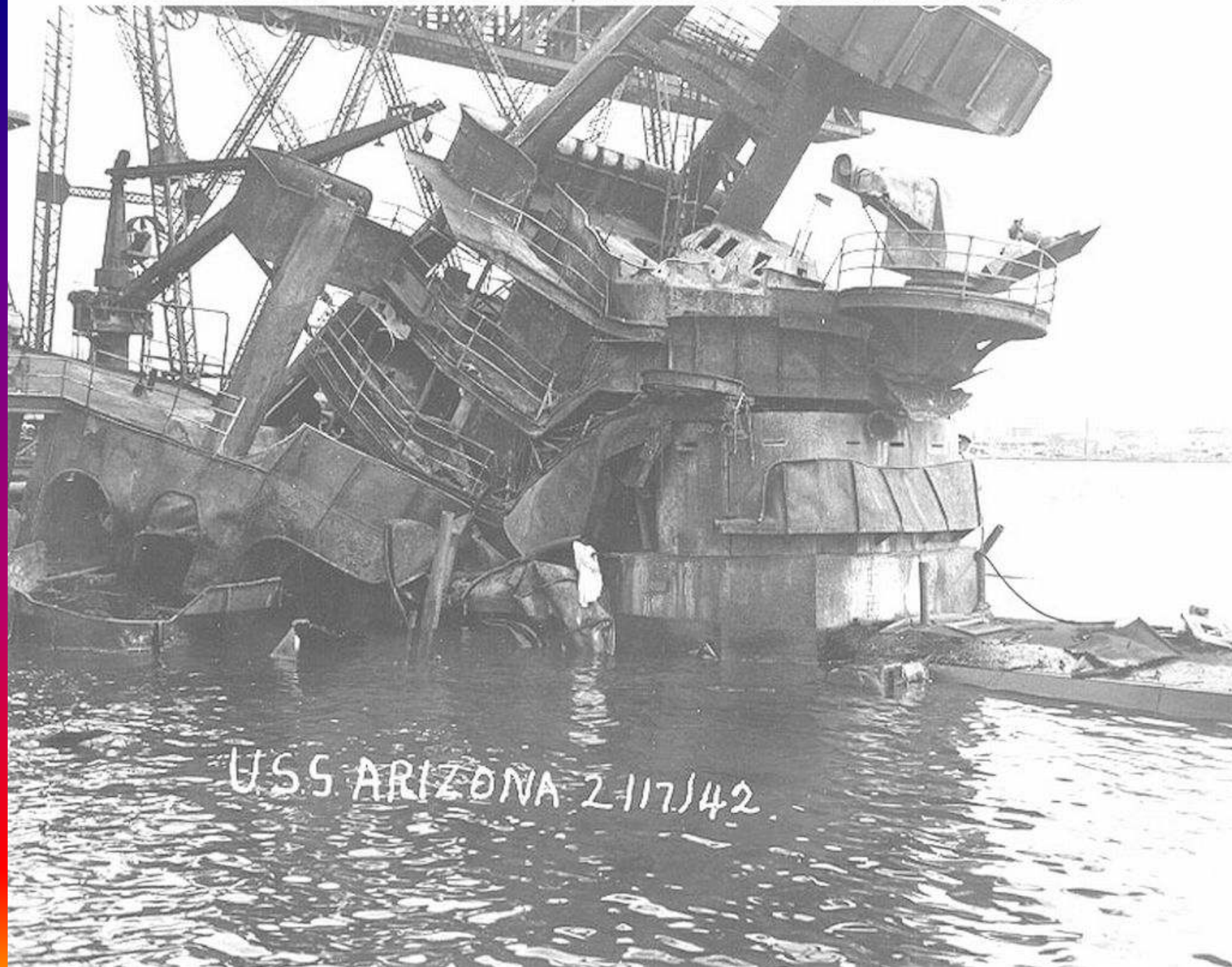
Photo # NH 83993 Wrecked forward superstructure of USS Arizona, 17 February 1942
